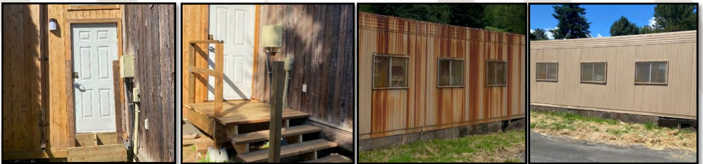
Xá:ytem site repairs.
