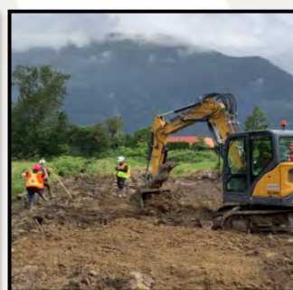
Machine excavation at Worth Road
